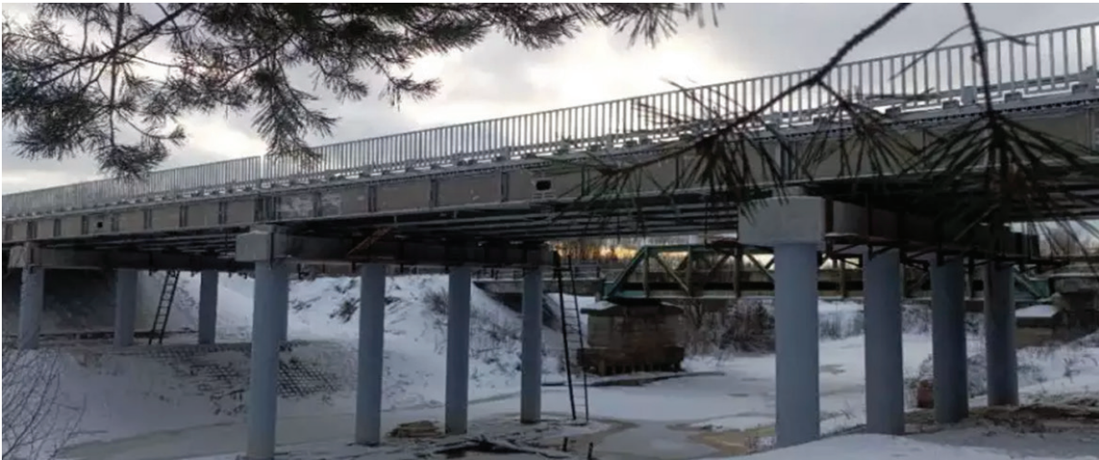
Fig. 4. Side view of the bridge, with the old single lane steel bridge visible in the background
