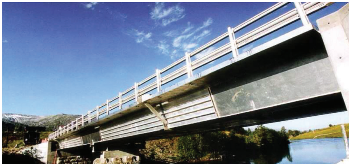
Fig. 2. Forsmo Bridge in Norway, span 39 m
