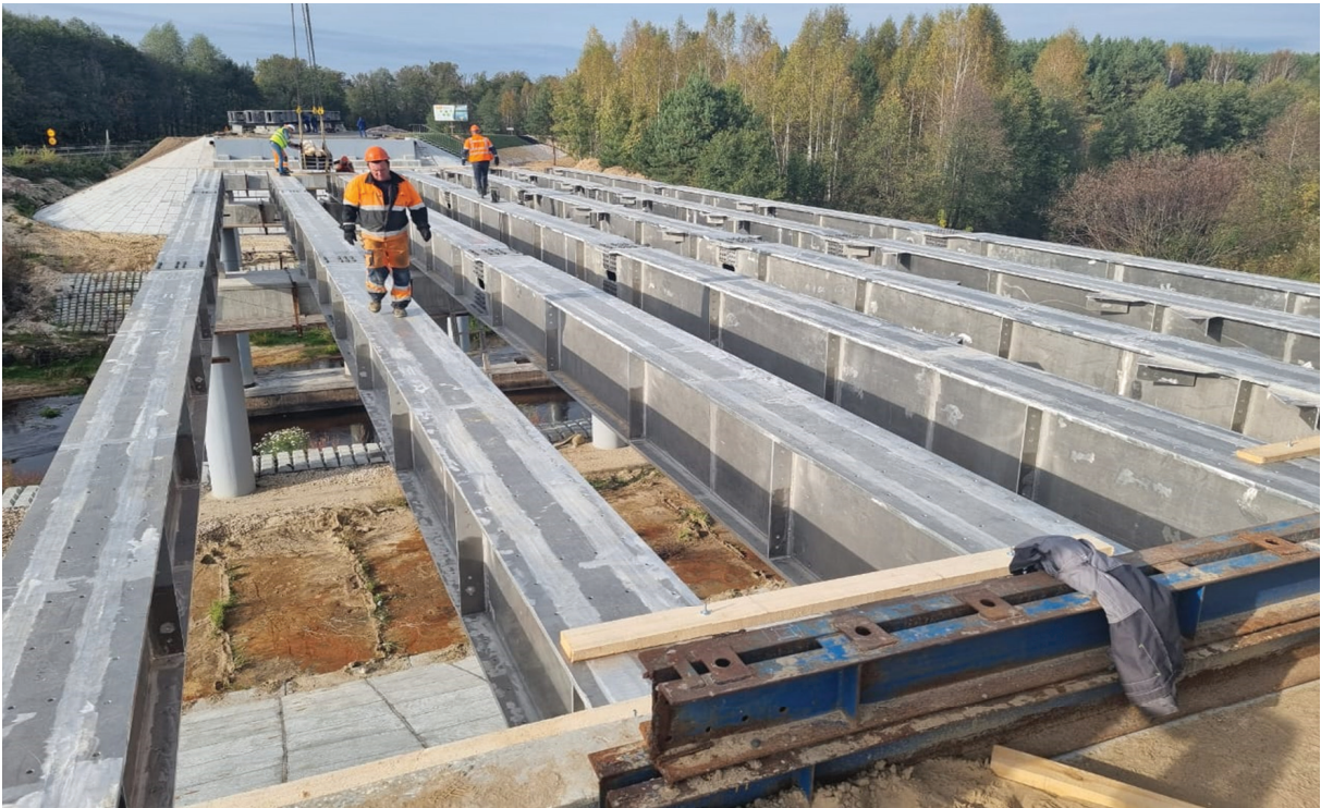
Fig. 18. Installed load-bearing girders of the span structure
