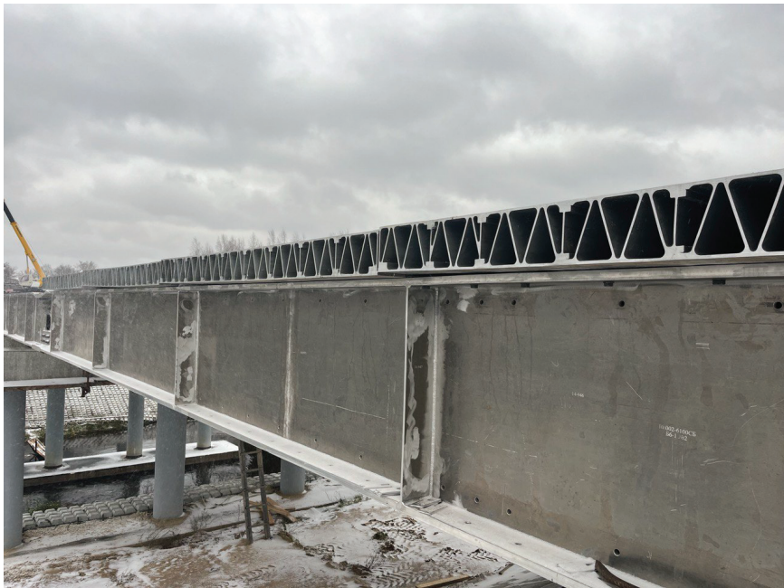
Fig. 19. Installation of orthotropic slabs on the supporting beams of the span structur
