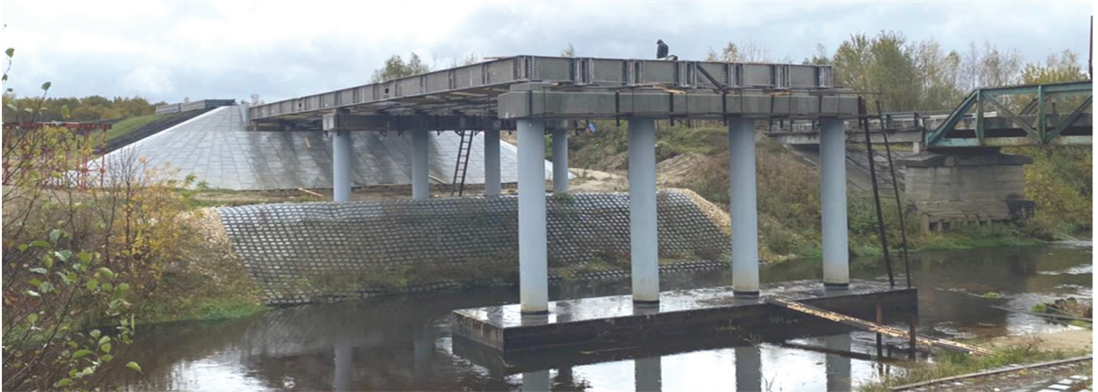
Fig. 17. Installation of the span on reinforced concrete supports
