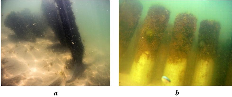
Fig. 4. State of the “Grebenka” breakwater modules: *a* – algae fouling and tilt of the structure (survey on 7 September 2022); *b* – post-storm partial exposure of the wave-damping piles from under sand (survey on April 12, 2023)
